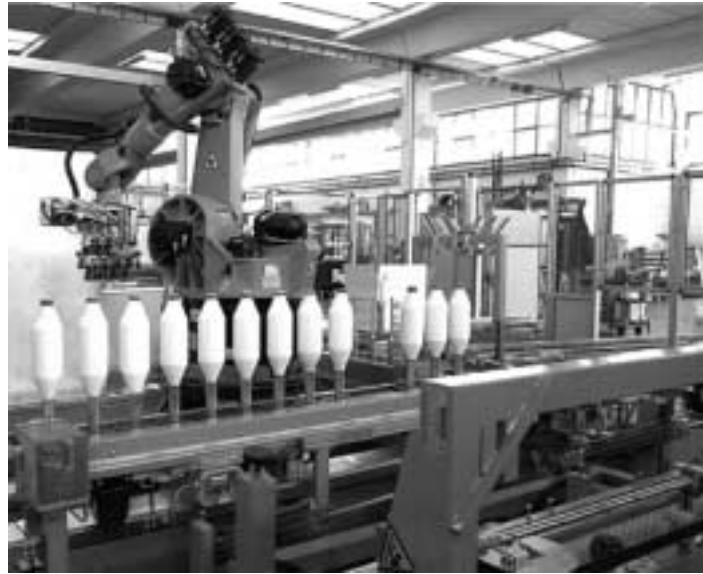
Fig. 68 – View of the handling and packaging robot
